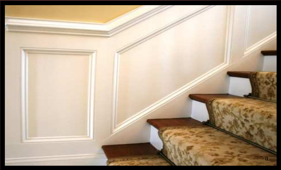
Wainscot Level 2 Recessed panels with sill +Chair 300
