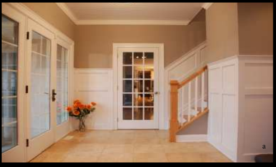
Wainscot Level 2 Recessed plain panels with Sill and ogee on top Double line
