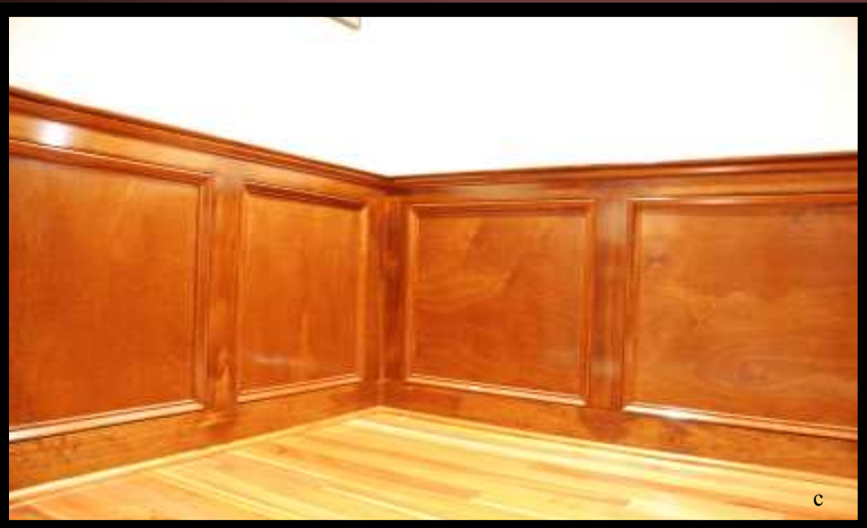
Wainscot Level 2 Recessed panels with Sill and ogee on top Stained Solid pine
