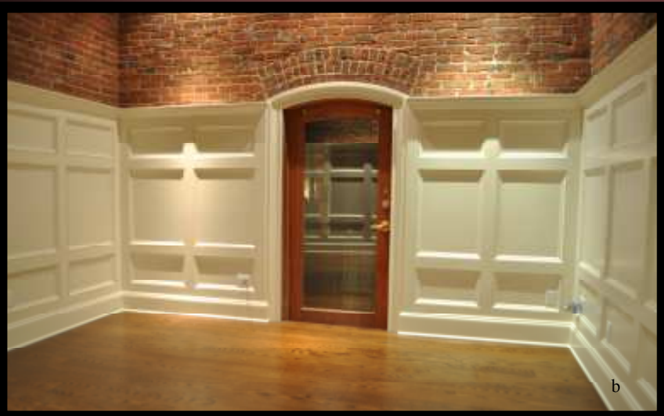
Wainscot Level 2 Recessed panels with Shelf and Crown on top Triple line
