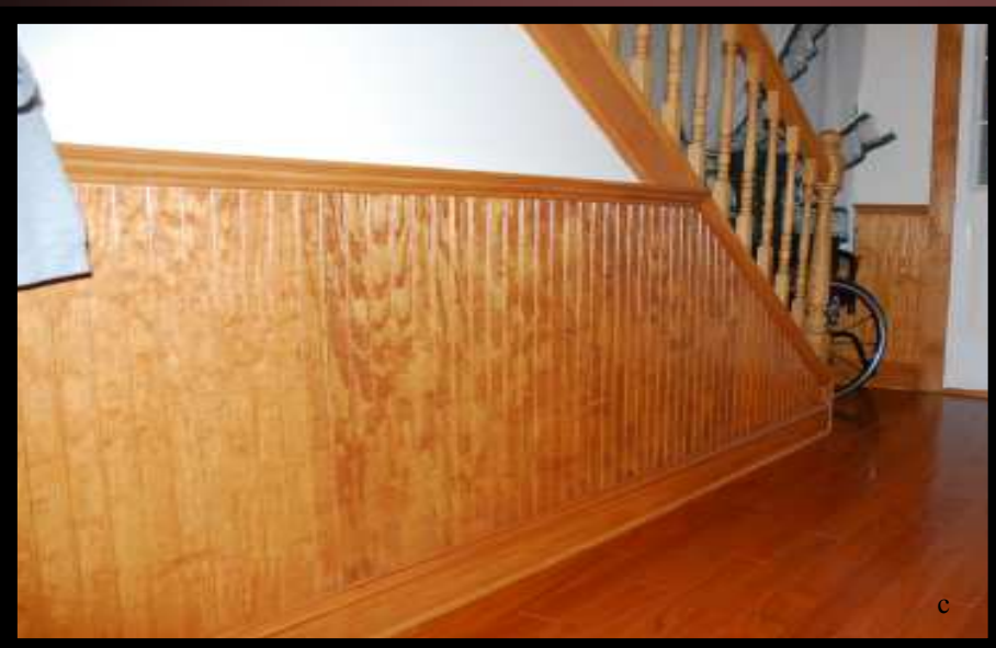
Wainscot Beaded Sill and ogee top Solid pine stained Base 5-1/4 163 solid pine
